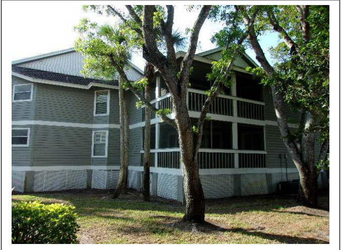
ROOF GEOMETRY – Other/Gable Roof Shape
