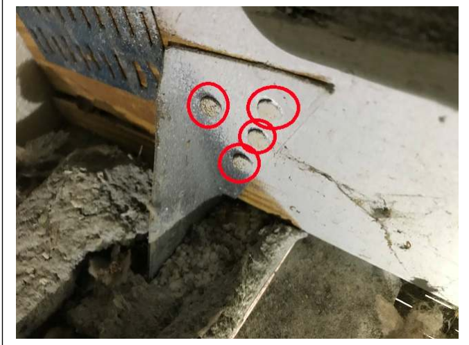
ROOF TO WALL ATTACHMENT – Properly installed Clips
