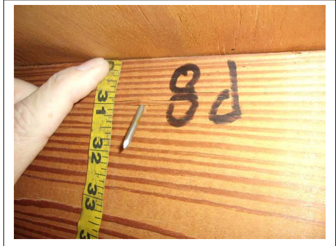
ROOF DECK ATTACHEMNT – 8d common nails added in 2006
