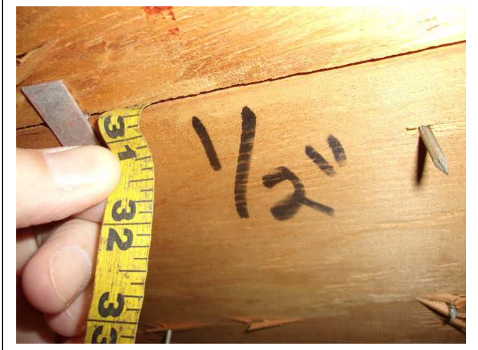
ROOF DECK THICKNESS – ½ inch plywood
