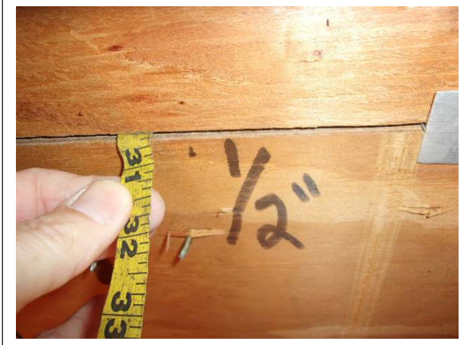
ROOF DECK THICKNESS – ½ inch plywood
