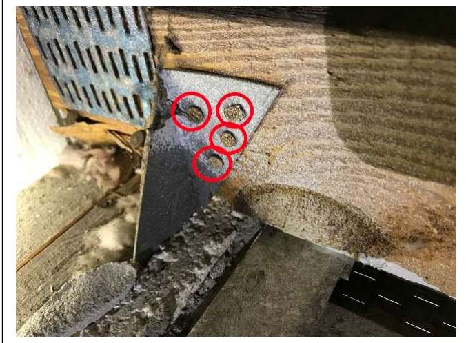
ROOF TO WALL ATTACHMENT – Properly installed Clips
